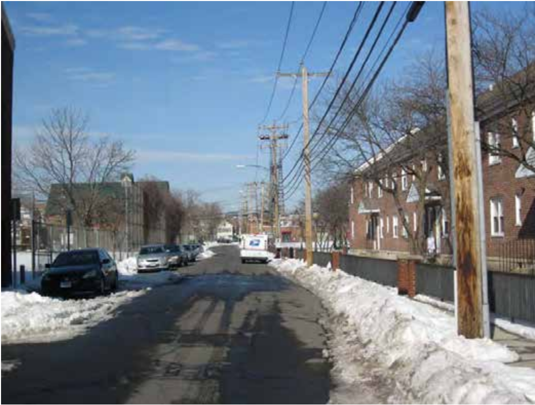
VIEW NORTH ON DAY STREET
