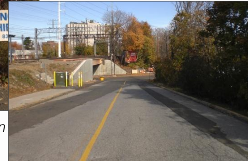
Lack of sidewalk connection EB Station to Monroe Street
