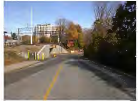
Eastbound Station – Looking North Toward Monroe Street Lack Of Sidewalks And Pedestrian Facilities
