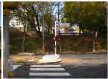
Lack Of Pedestrians Ramps Crossing MLK At Madison Street
