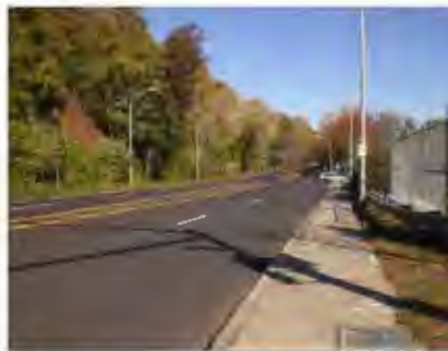
Lack Of Pedestrian Refuge Island On MLK At Spring Street Requires Pedestrians To Cross Four Lanes Of Traffic
