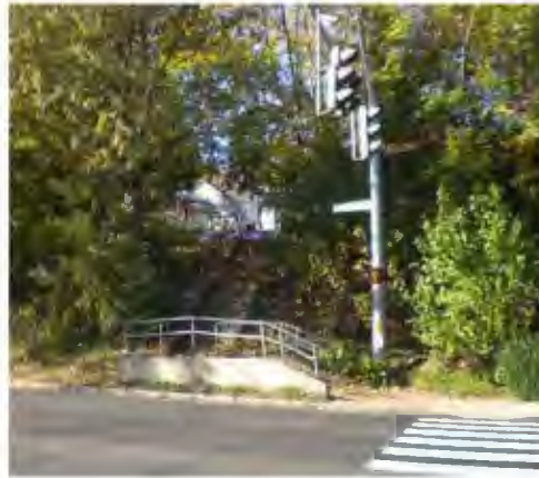
Stairway At Spring Street Leading To Hamilton Avenue
