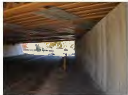
Railroad Overpass On Monroe Street Creates A Dark And Unappealing Environment
