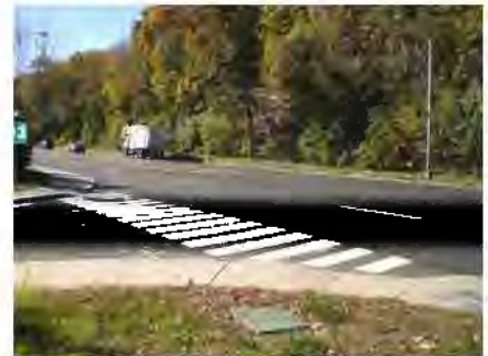
Westbound Station – Looking South On Dr. Martin Luther King Jr. Drive: Large Turning Radii Encourages High Automobile Speeds And There Is Limited Visibility For Pedestrians At The Entrance
