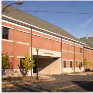
Water Street (left): Primary Street Monroe Street (right): Connector Street
