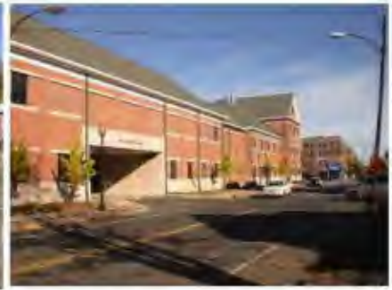
Well-Maintained Sidewalks And Streetscape Amenities On Monroe Street Along The Frontage Of The Police Station
