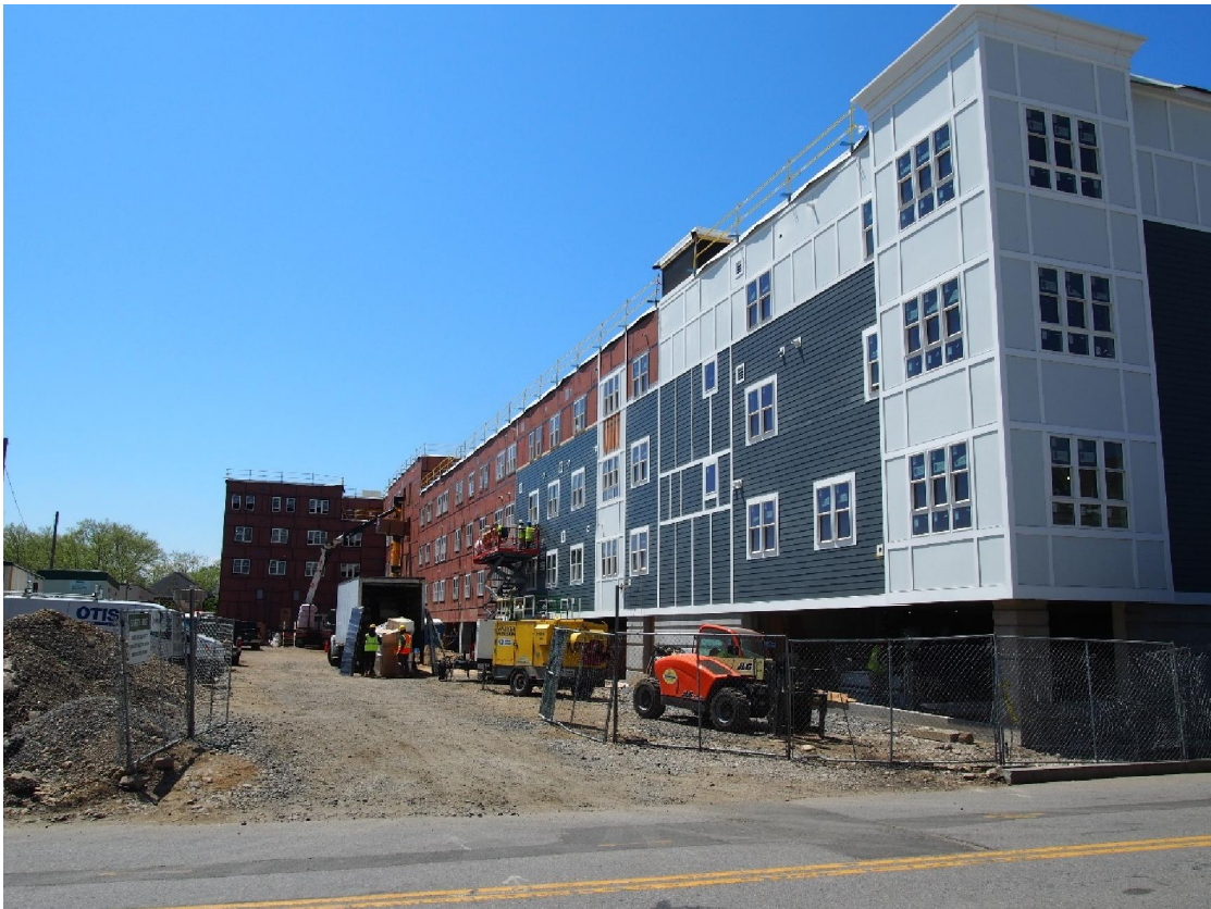
East Elevation of 20 Day Street
