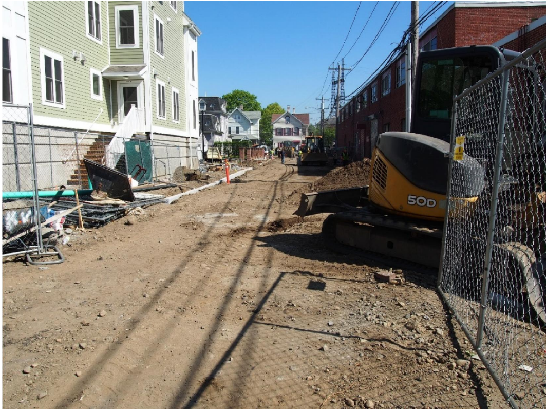
Day Street Extension – Hanford Place to Elizabeth Street
