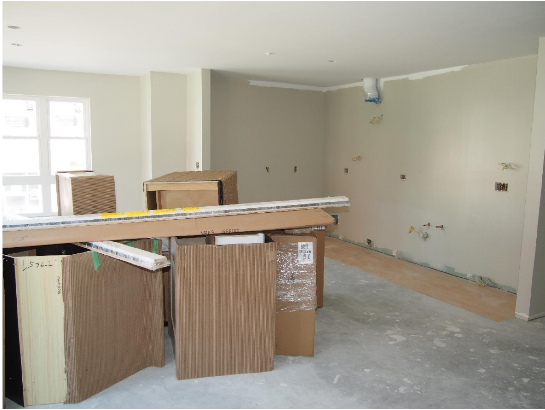
Painted Apartment with Kitchen Cabinets ready for Installation
