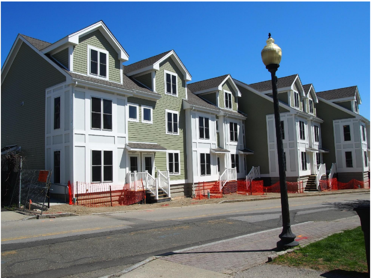
Building A, 13 Day Street
