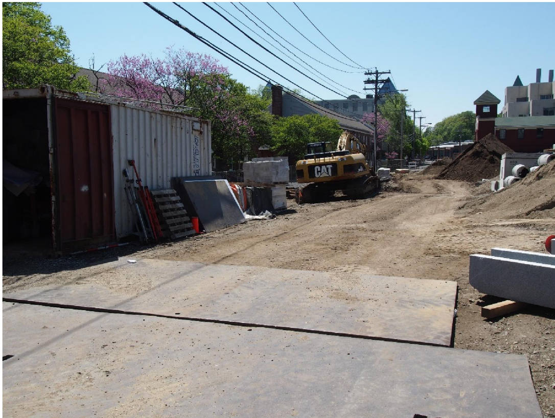
Looking South on Day Street
